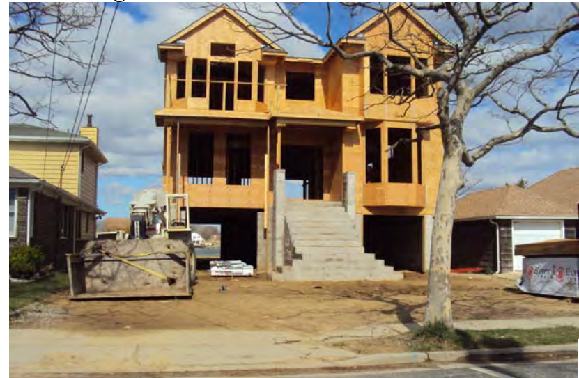
Figure 12: New Home under Construction
