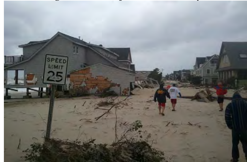
Figure 8: Sand Deposited on Roadways
