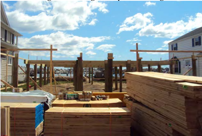
Figure 11: Pilings Ready for Framing
